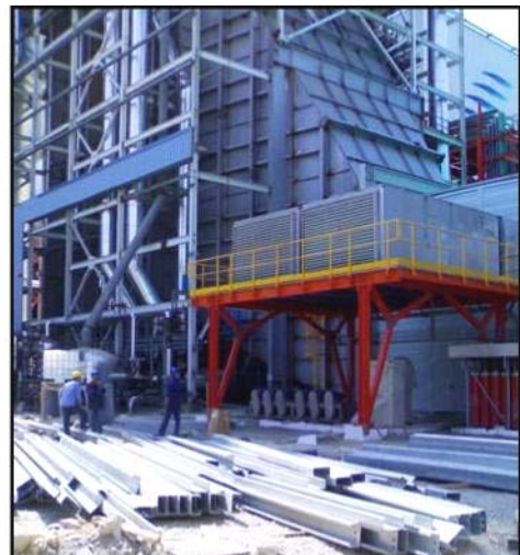
Pump Skid Installation next to the Air Intake at Vado Ligure
