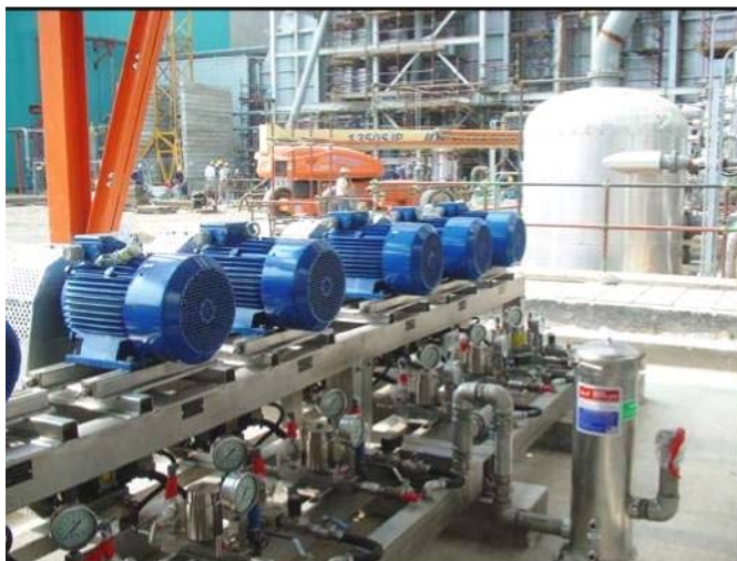
Pump Skid Installation next to the Air Intake at Vado Ligure
